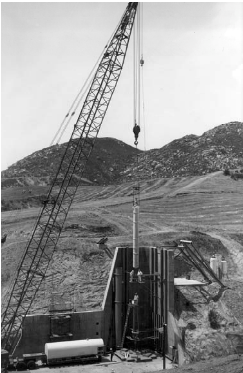
Figure 14. Booster is removed from conditioning cell in preparation for a cold static test.
