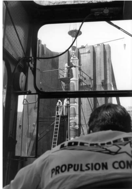
Figure 17. Crane operator's view.
